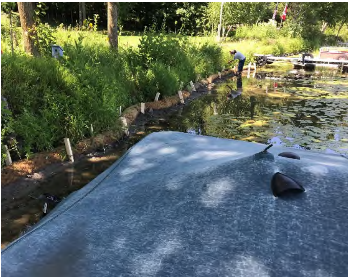
Coir Log after install
